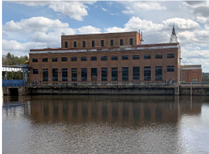
Heavy turbine leakage was causing issues.
